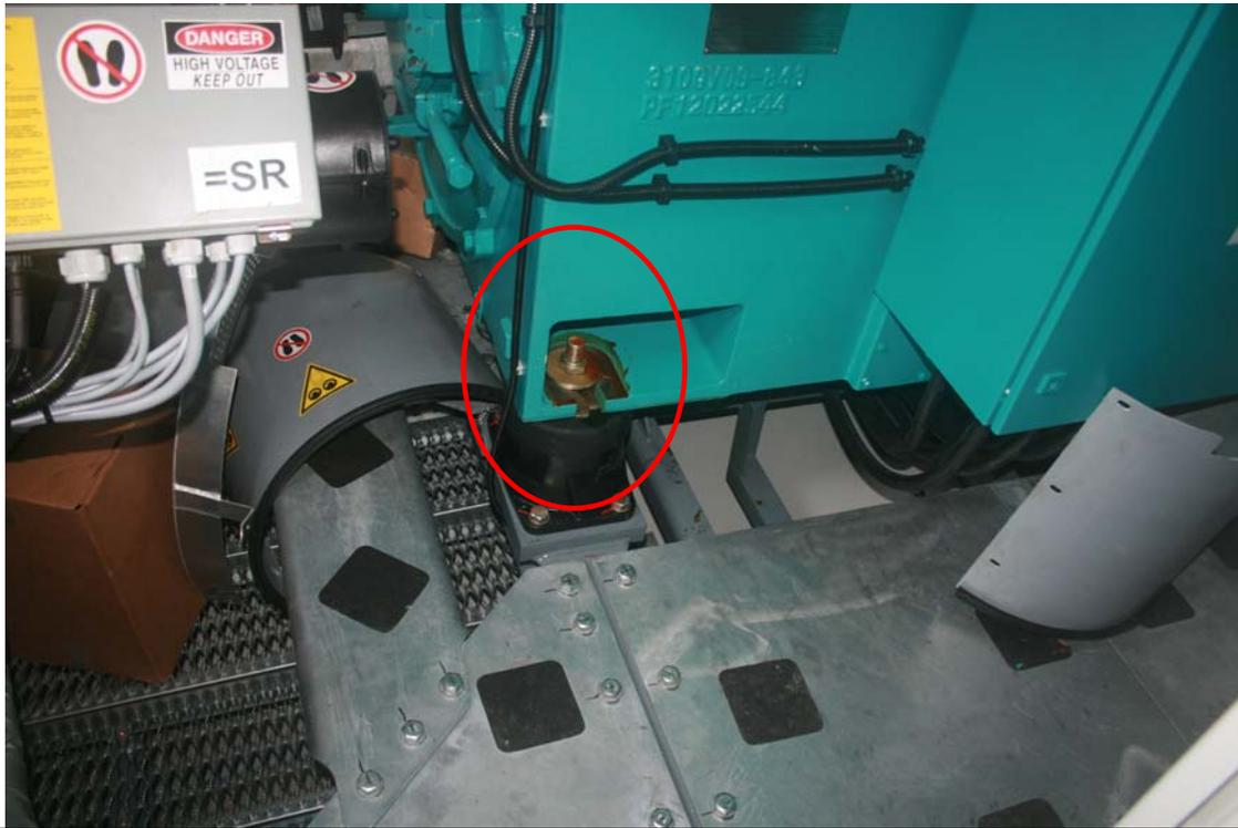
Figure 35 Left front generator mount.
