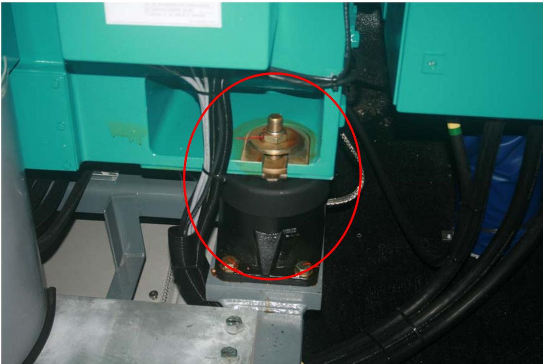
Figure 38 Left rear generator mount.
