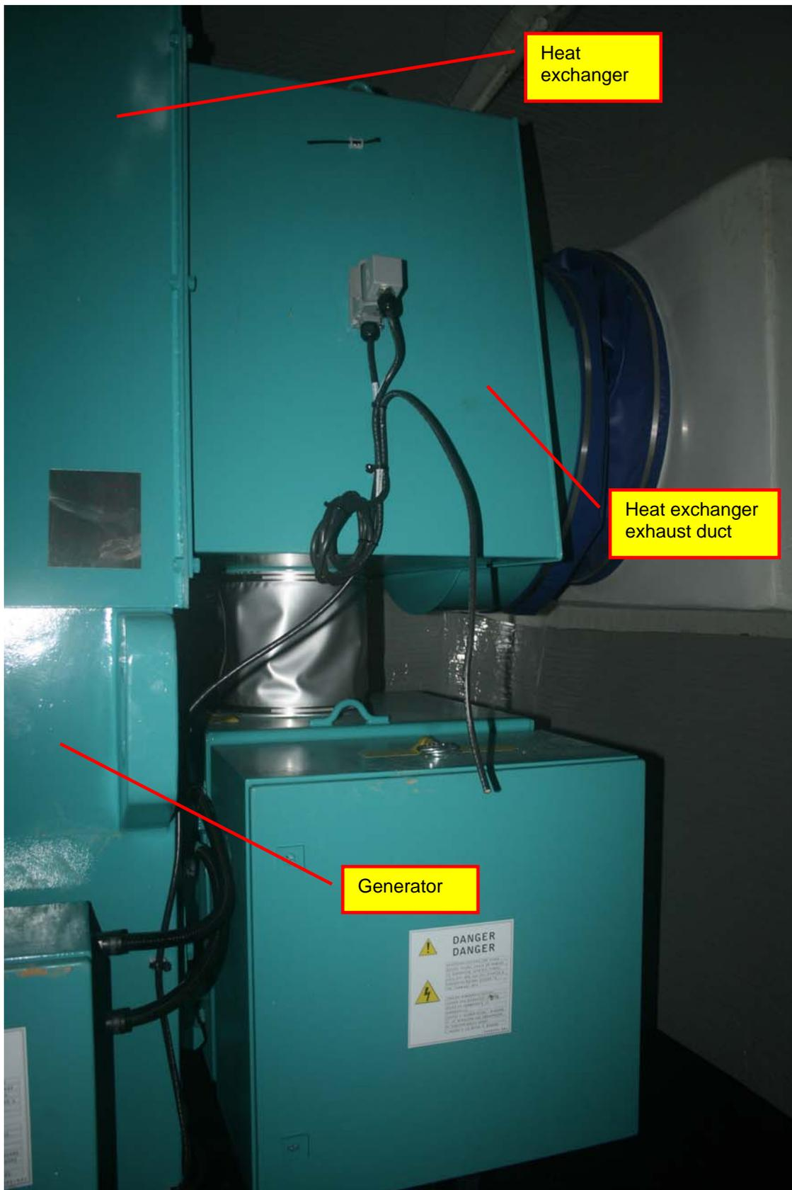
Figure 12 Aft end of generator with heat exchanger discharge duct through nacelle; viewed from the right side.
